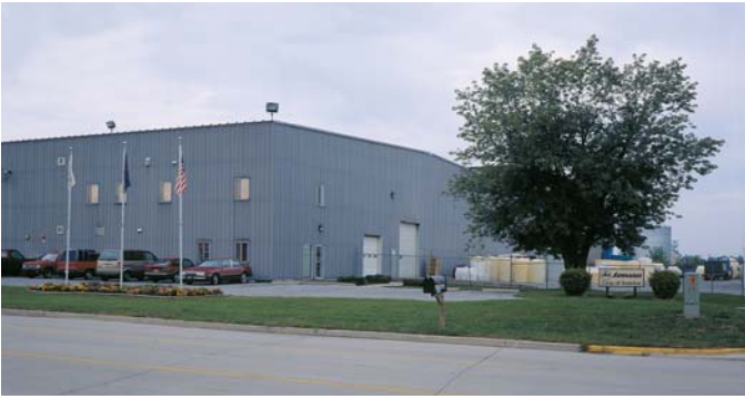
Garrett, Indiana Facility
